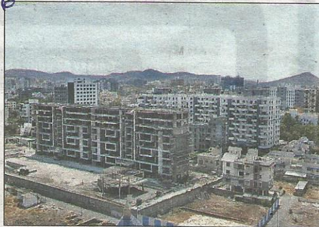
100 plus buildings have no completion certificates.
